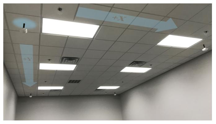
Note: the above images show the Anchors installed in a ceiling grid. Users unfamiliar with system operation may wish to place Anchors on a tripod in an open area to gain familiarity with the system before doing a more permanent installation
